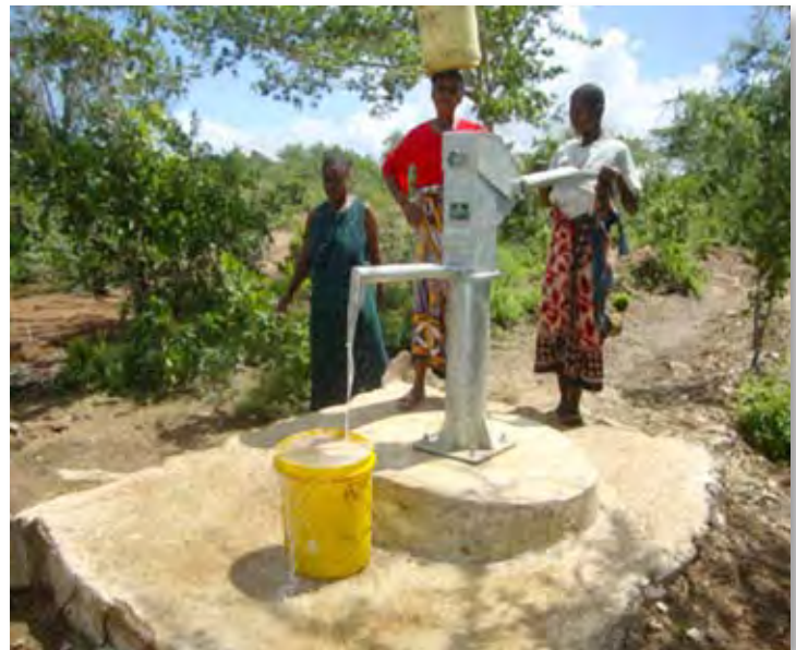
COMMUNITY EFFORT: Mariam Milton Zuma and other women in Mabesheni Village, Kinango District, Kenya draw water from a filtration gallery installed at a community-managed small farm reservoir fitted with a hand pump.
