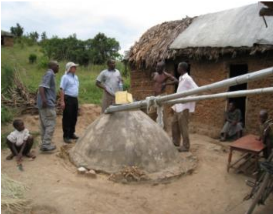
Figure 4.8 Partially below ground tanks in Isingiro District
