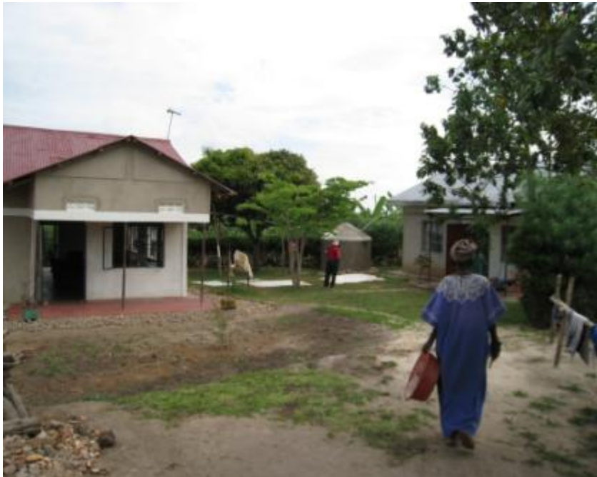
Figure 4.3 DRWH Facility Constructed with Support from the DWSCG in Bushenyi District Local Government
