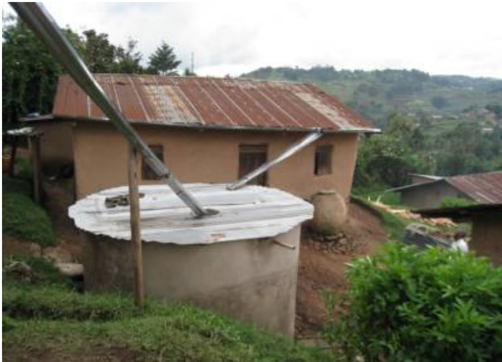
Figure 4.10 Facilities upgraded from a 420 litre jar to a 4m 3 tank in Muko, Kabale District
