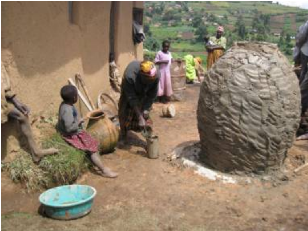
Figure 4.9 Upgrading from a Clay Pot to a Ferrocement Jar in Kabale District
