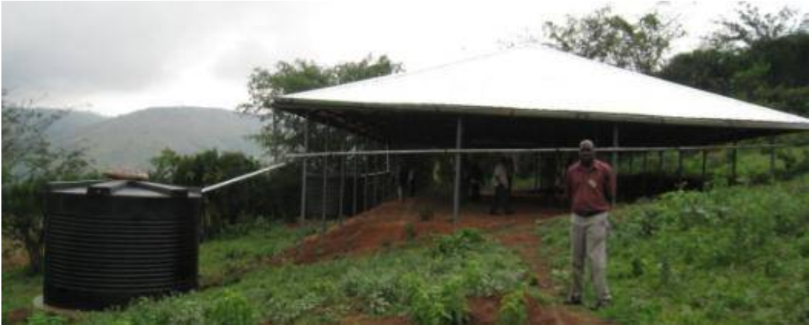
Figure 2.8 Community Rainwater Harvesting Facility in Masaka District
