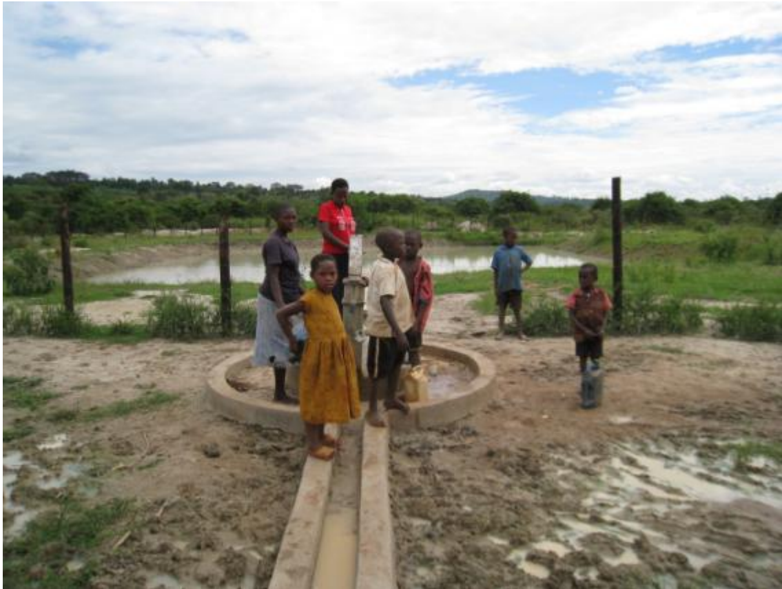
Figure 2.5 Valley Tank with Handpump in Masaka District
